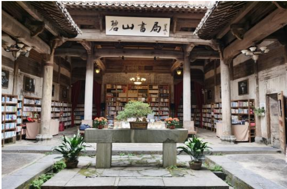
Fig.8 The drainage of the patio
