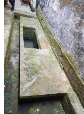
Fig.9 The drainage of the patio
