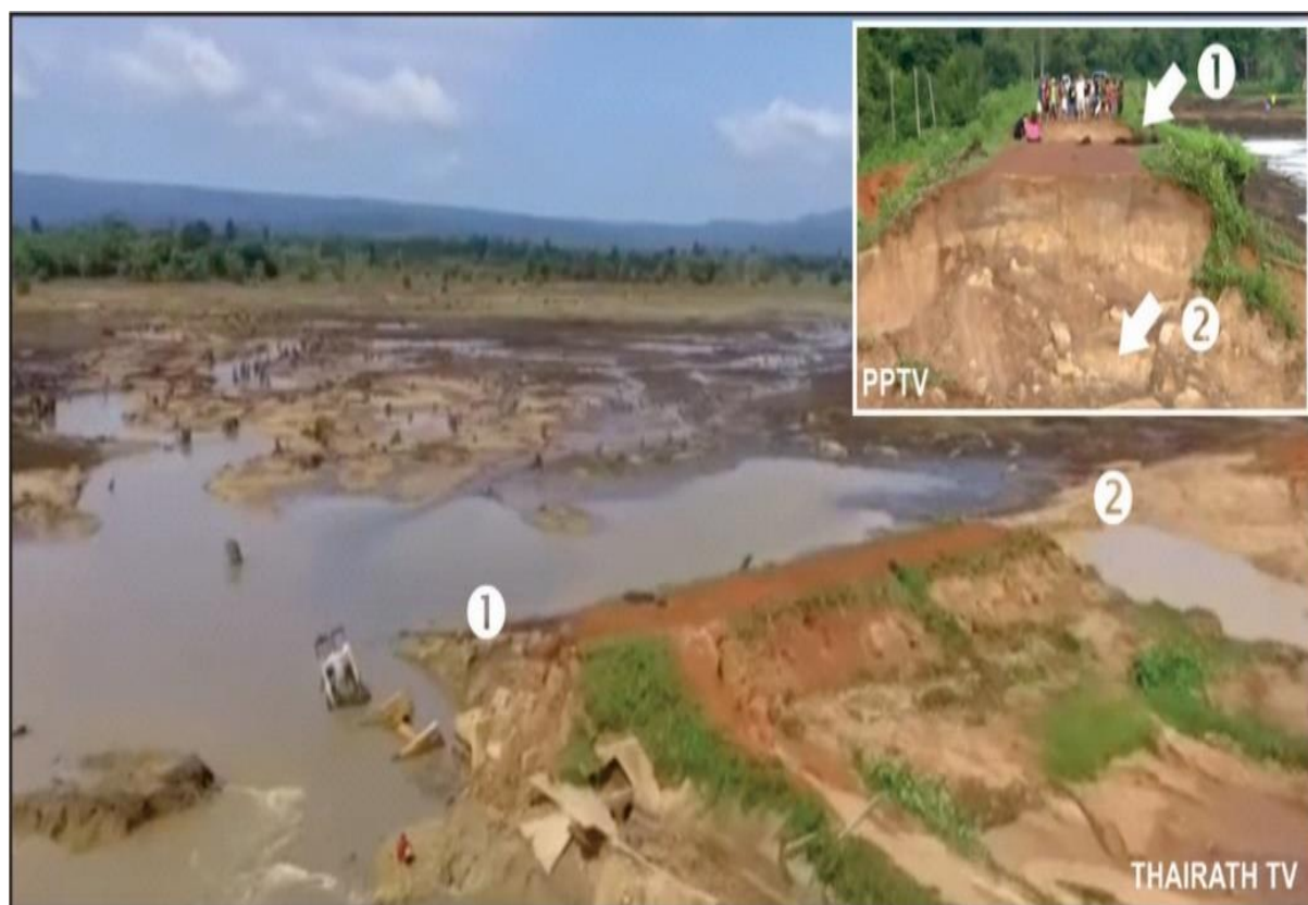
Figure 4 An aerial view showing the two breached sites of the Huai Sai Kamin embankment, one site at the left water gate and about 25 meters away from the other site. An insert photo shows embankment cross section in the opposite view [11,18].
