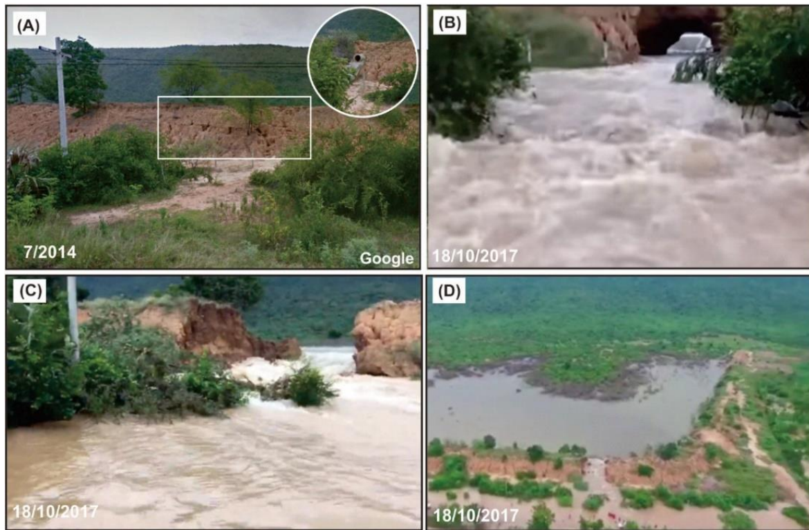
Figure 2 (A) Photograph of the embankment of the Nong Sano reservoir taken in July 2014 from Google Map, a square box outlined an approximate breached location that occurred in October 18 th , 2017, an inserted photo showing a conduit installed for water outflow as water in a reservoir exceeds the maximum capacity [13], (B) and (C) photographs captured from video clip taken during the failure incident, showing an internal erosion through dispersive soil [14], (D) an aerial view showing a breached location and water in the reservoir [14].
