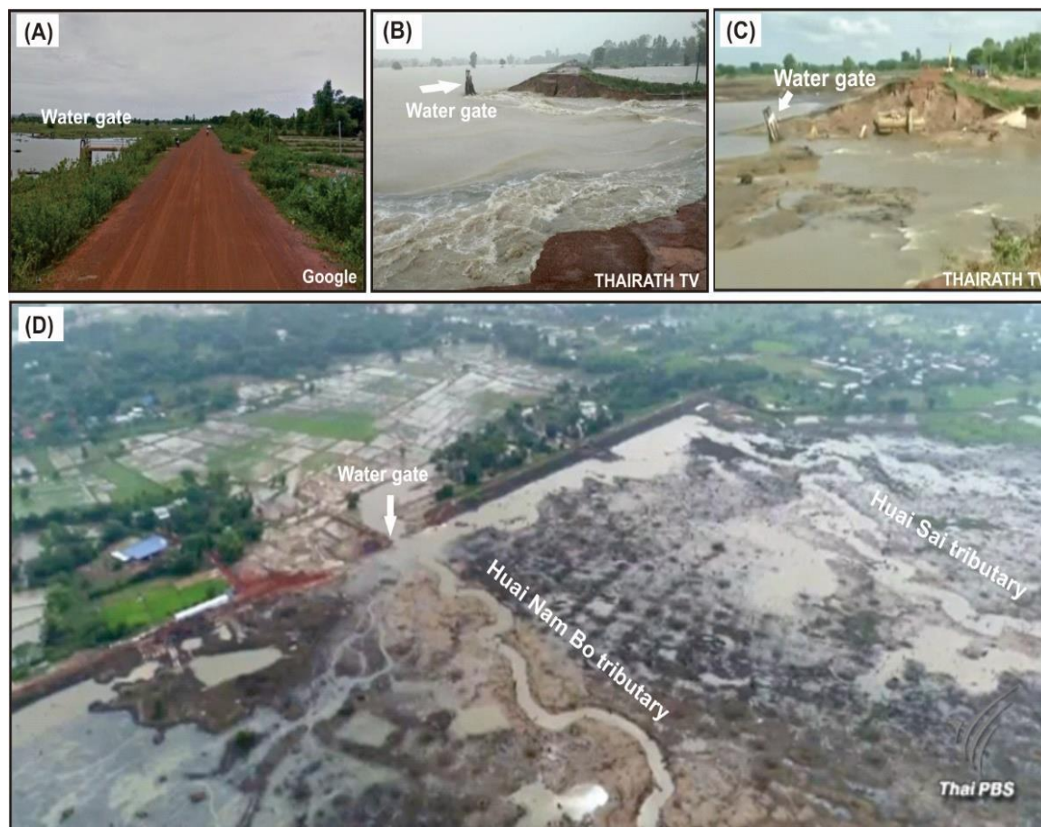
Figure 1 (A) Photograph of the Huai Sai Kamin dam taken in June 2015 from the Google Map showing the embankment crest, fillings in the reservoir and the water gate where the left conduit installed beneath the embankment [9], (B) and (C) photographs of the dam taken in the morning and in the afternoon of July 28 th , 2017 after a breach incident occurred, the water gate shown in (A) was collapsed [10-11], (D) an aerial view taken on July 31 st , 2017 showing the dam no longer held water and the remnant of Huai Nam Bo tributary that ran through the embankment [12].
