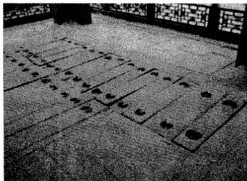
Fig. 15 a. The pathway to the underground covered with the “movable covered boards” on the Longevity Stage. Photo taken inside the Longevity Stage of the Pleasant Sound Pavilion by Sasiporn Petcharapiruch on November 11, 2004.
