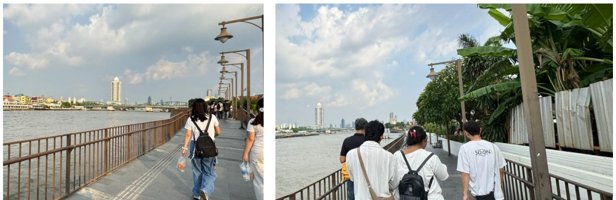
Figure 8 Riverside Promenade. (Left) Lack of shade along the walkway; (Right) privacy screening and walls along the walkway
