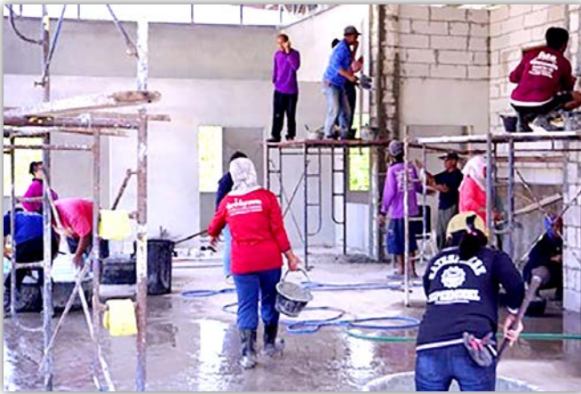
Figure 5 Practical training course on constructing a light brick wall and practical test
