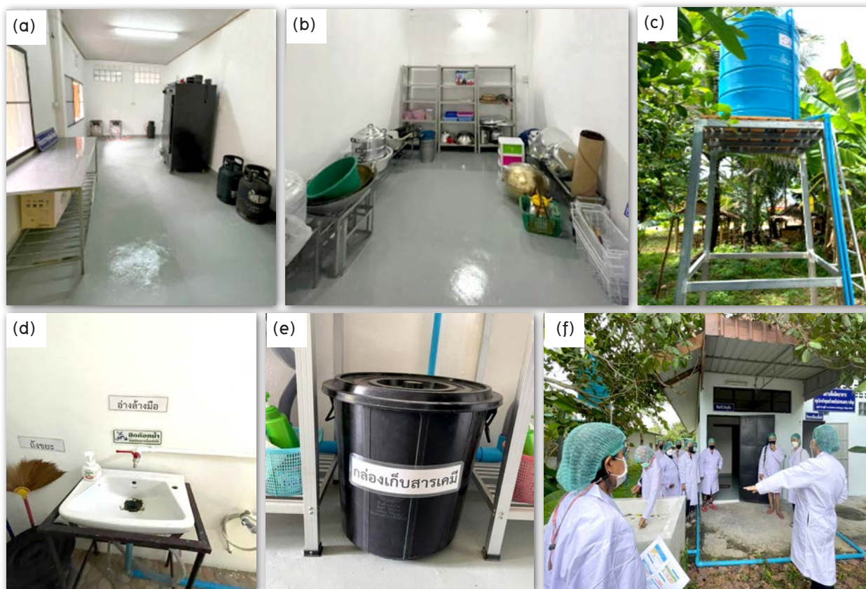
Figure 6 Improvement of food production processes; (a) Organizing the production workflow, segregating packaging areas to prevent contamination, and improving building floors to be even and free from dust and pathogens, (b) Providing additional equipment necessary for the production process, and organizing items neatly, (c) Installing water reservoirs to rinse raw materials and equipment to meet standards, (d) Providing an adequate supply of hand soap at each handwashing station, (e) Storing cleaning chemicals proportionally and clearly labeled points of chemical storage for cleaning purposes, and (f) Conducting training sessions to educate employees about hygiene
