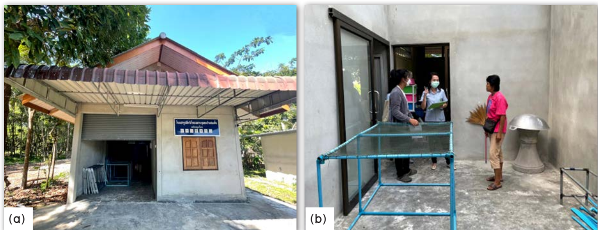
Figure 5 Processing facility; (a) Outside and (b) Inside
