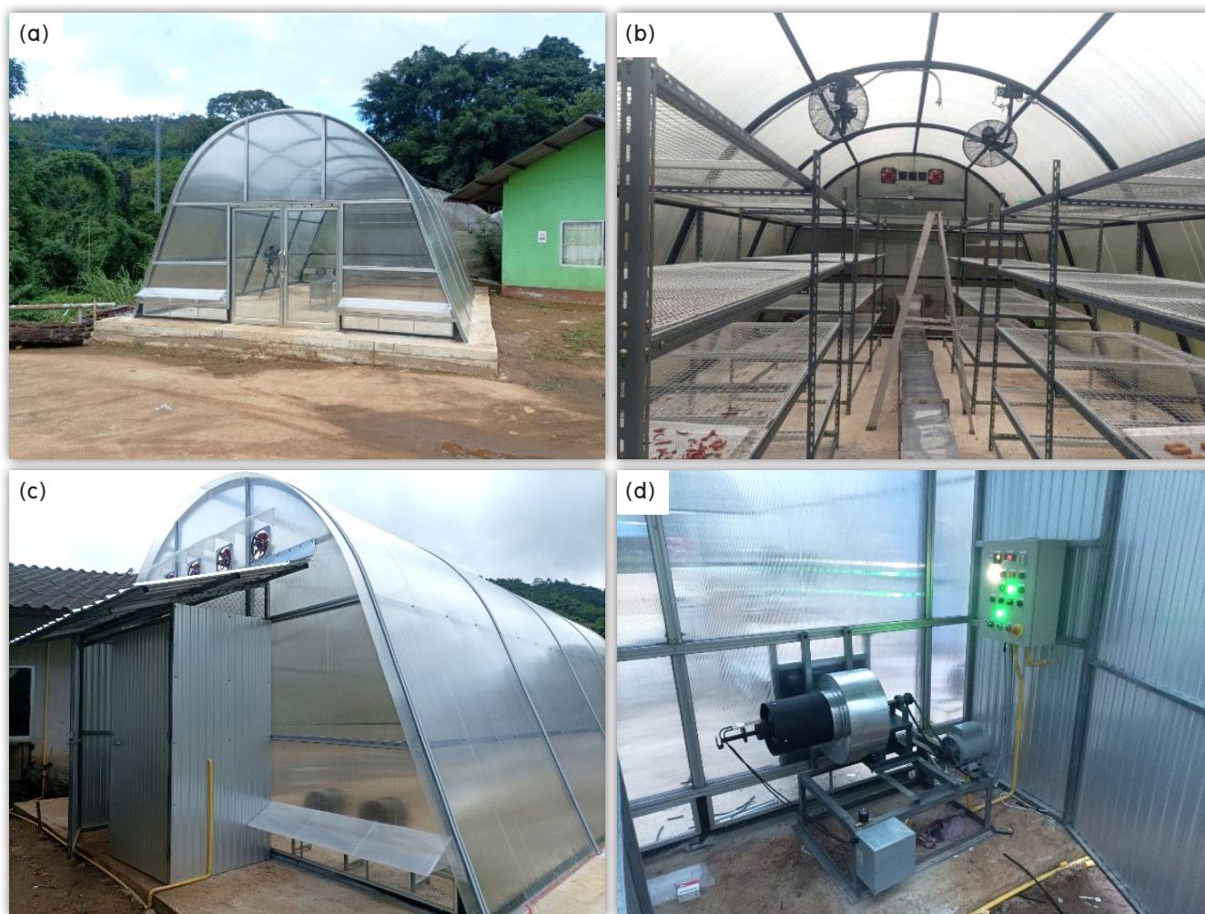
Figure 7 (a) Greenhouse solar dryer, (b) Inside greenhouse solar dryer, (c) Control room, and (d) Supplementary heat airflow system
