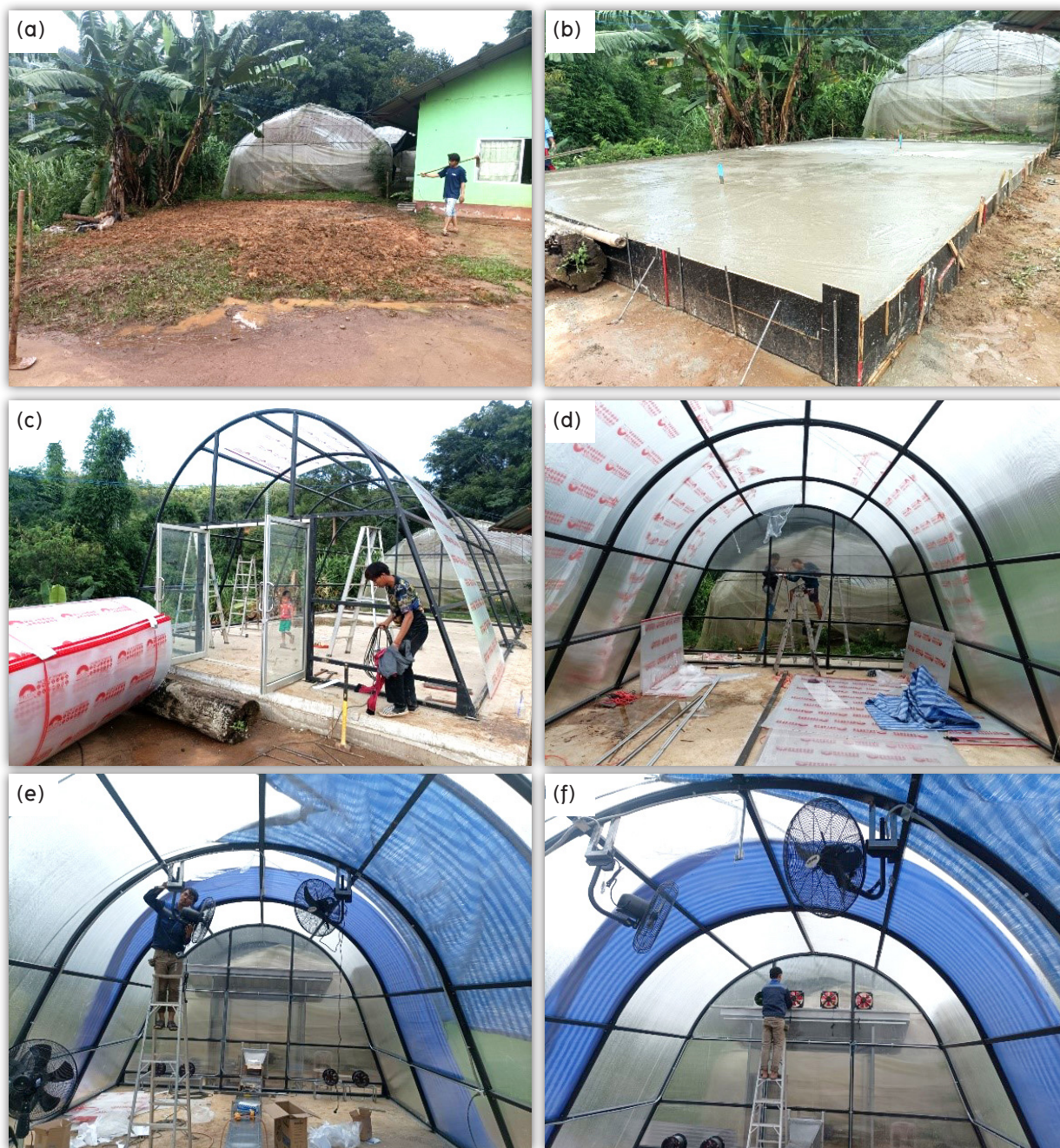
Figure 6 Steps to Install a greenhouse solar dryer with automated control for supplementary heat and airflow; (a) Area preparation, (b) Cement base construction, (c) Installation of solar dryer structure, (d) Polycarbonate wall installation, (e) Ventilation fan installation, and (f) Exhaust fan installation
