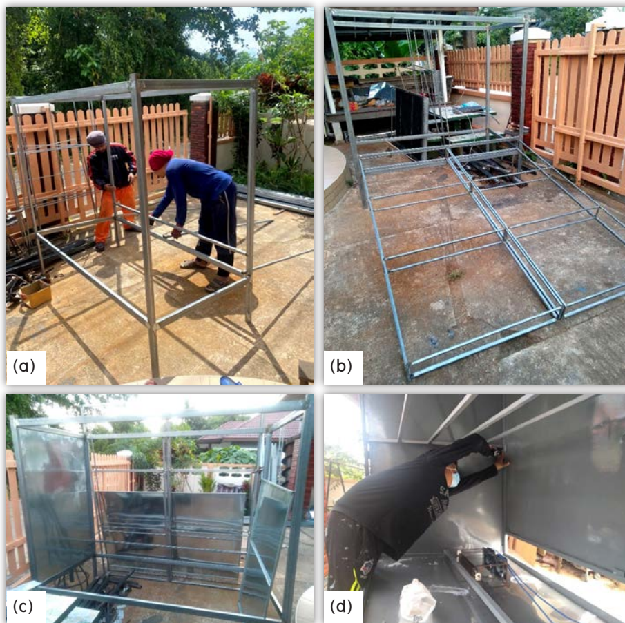
Figure 5 Passive solar drying system; (a) Welding and assembly of the drying chamber, (b) Welding and assembly of the drying chamber frame with the solar collector, (c) Installation of the chamber walls, and (d) Installation of racks for hanging salted four-finger threadfin inside the drying chamber
