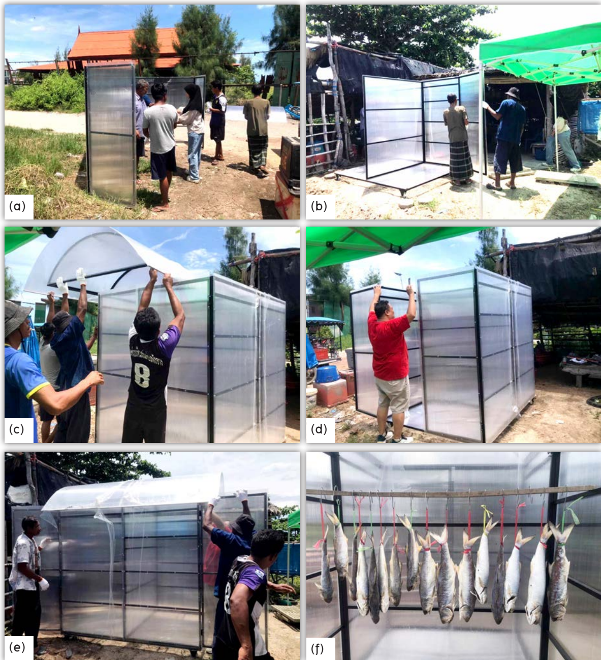
Figure 5 Installation of solar drying cabinet; (a) Components of solar drying cabinet, (b) Installation of the base and cabinet partitions, (c) Assembly of the side wall, (d) Roof installation, (e) Inspection for vulnerabilities and detail collection, and (f) Fish drying experiment using solar drying cabinet
