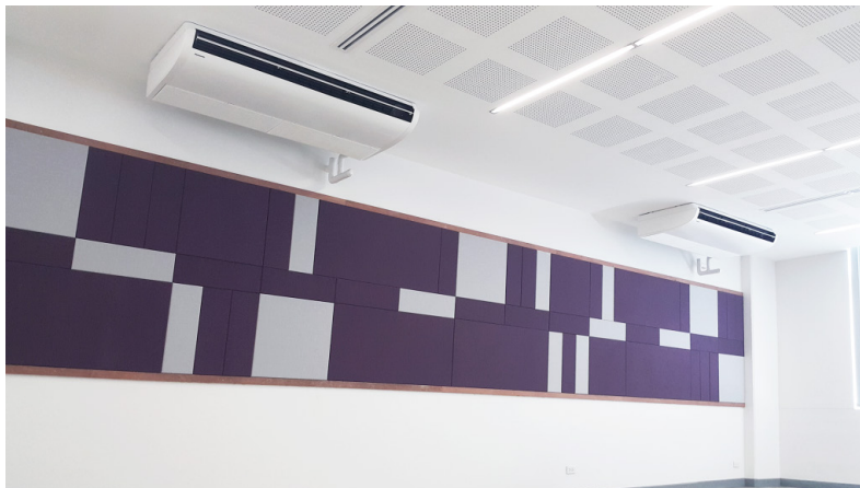
Figure 13 Air conditioner positions and sound-absorbing material installation after interior finishing
